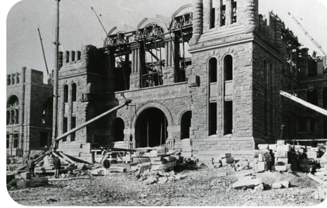
Construction on the interior and exterior walls in 1887. The interior walls are made up of over 10 million red bricks.
