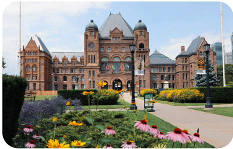
Richardsonian Romanesque architectural features include heavy rock-faced stonework, intricate designs, rounded archways, and turrets.
